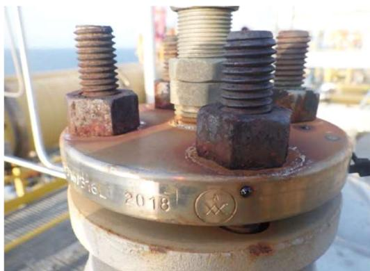
By changing out corroded or degraded bolts whilst production continues, there is a reduction in the workload carried out during an upcoming shutdown.
